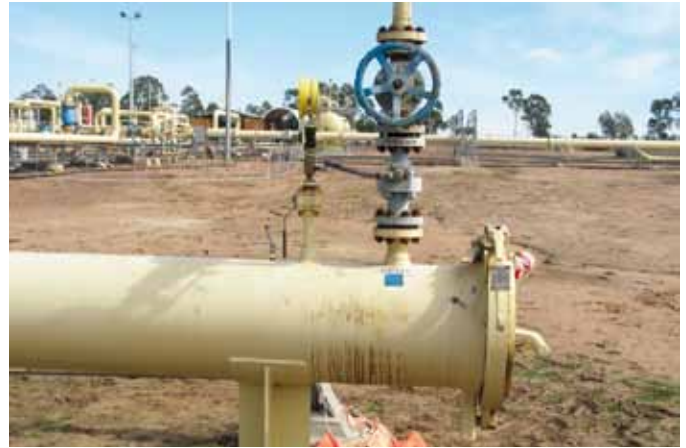
Pig receiver and sampling point
