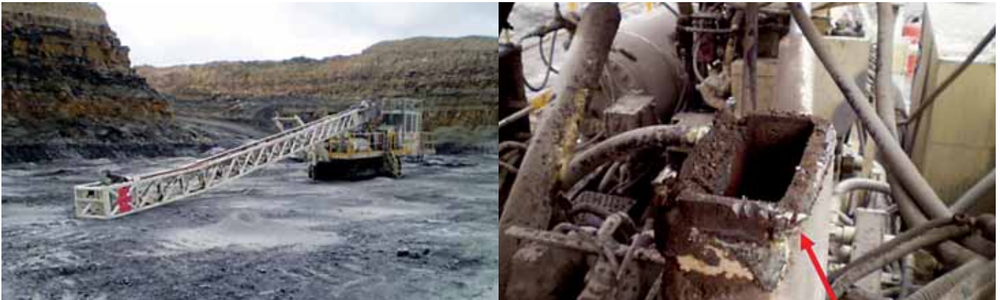
The collapsed drill rig mast (left) and the drill rig's failed pivot point (right) on the RHS tubing.
